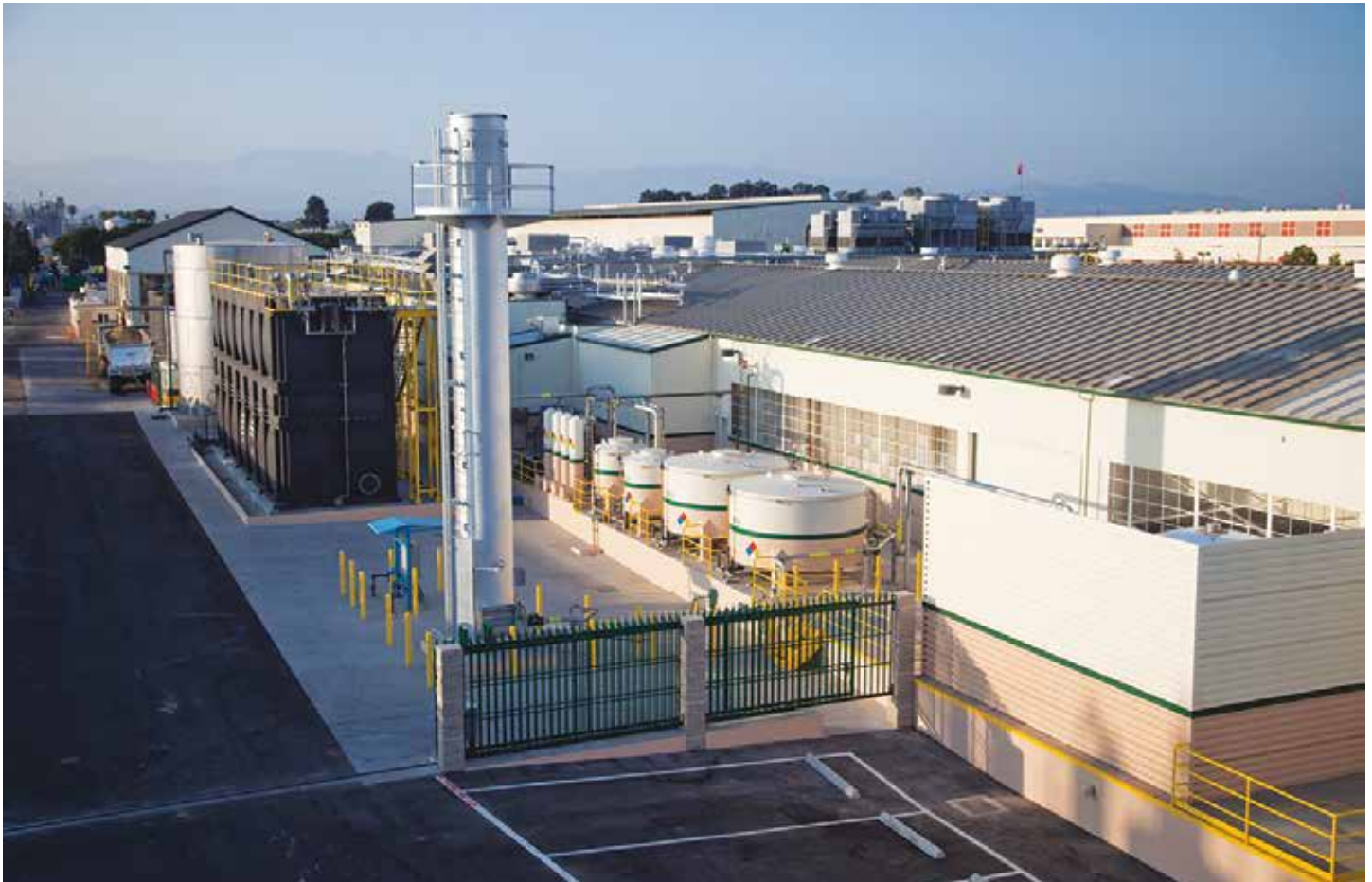
Gills Onions' Advanced Energy Recovery System converts onion waste into electricity
